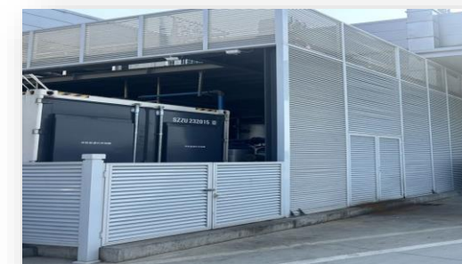
Noise source isolation measures
