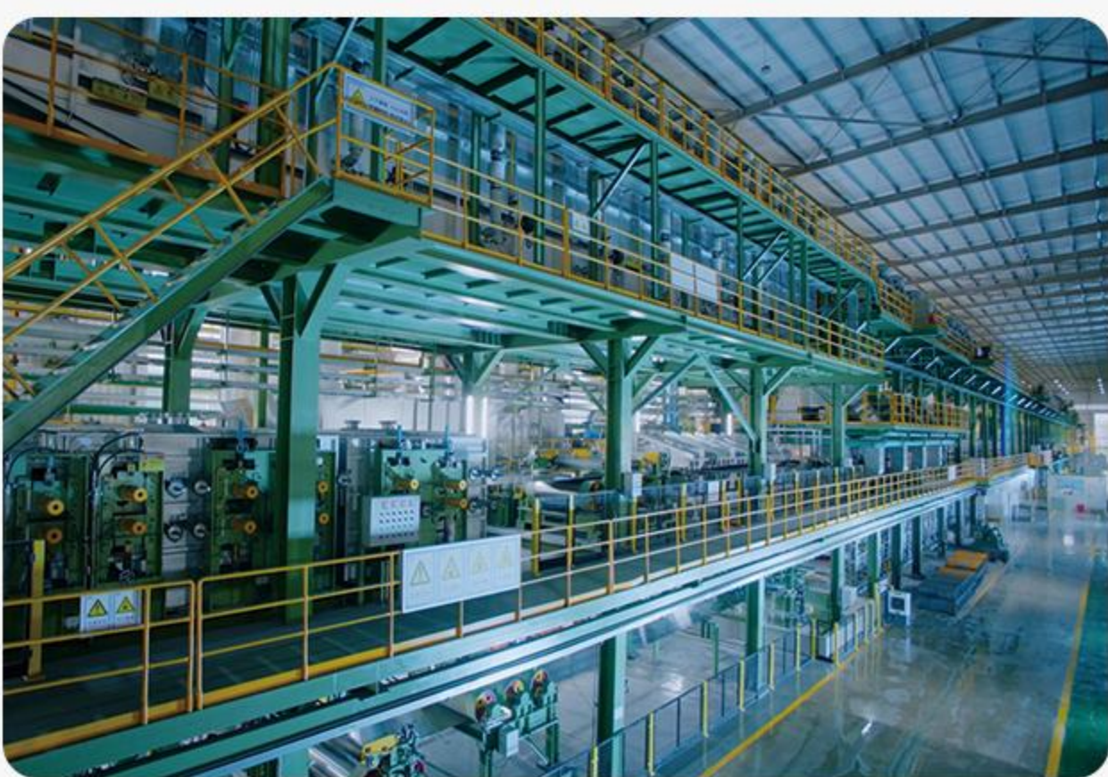
Pioneering CA and CT production lines Multi-layer stacked factory design
